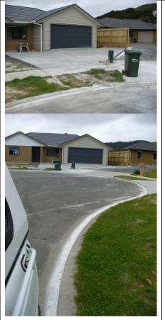
Exposed aggregate wash runs into gutter and stormwater. Note instructions for correct use are stated on container label. It clearly states to prevent wash getting into stormwater or waterways.
