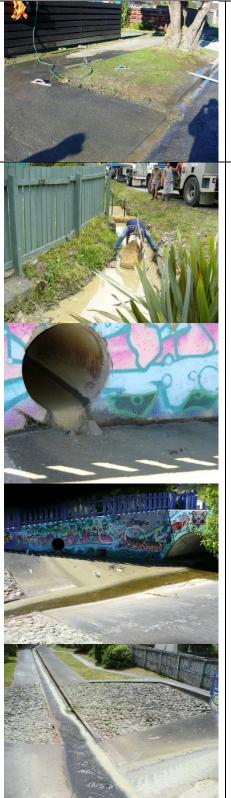
Clean up after concreting washed into gutter and stormwater.
